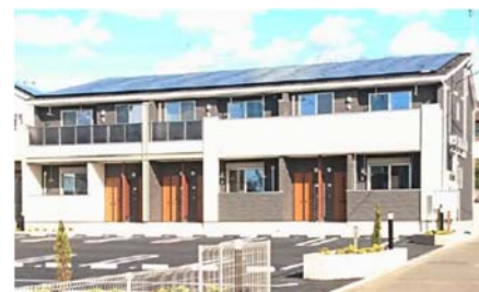
ZEH multifamily rental apartment provided by the Daito Group
