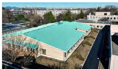
Palliative Care Ward, National Hospital Organization Tokyo National Hospital
