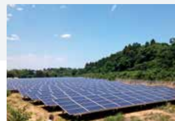
Yamato Ibaraki No. 2 Power Plant
