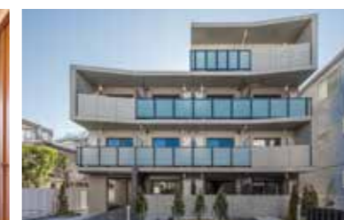
Exterior of special-order building
