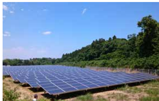
Mega solar plant
