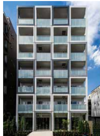
Exterior of special-order building
