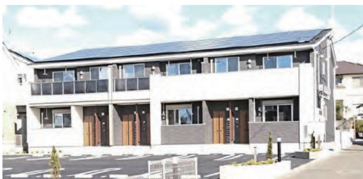
A building being constructed using 100% renewable energy
