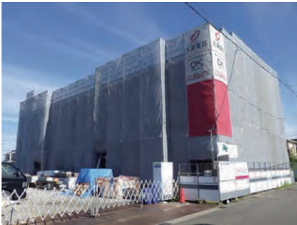
A building being constructed using 100% renewable energy
