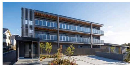
Three-story rental housing product by adopting our proprietary CLT construction method “Forterb III”
