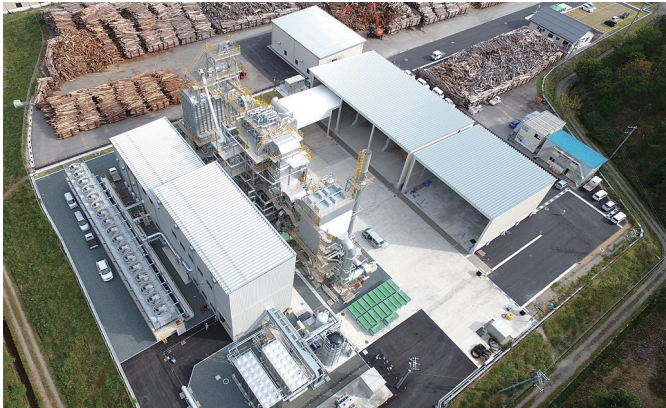
Asago Biomass Power Station
