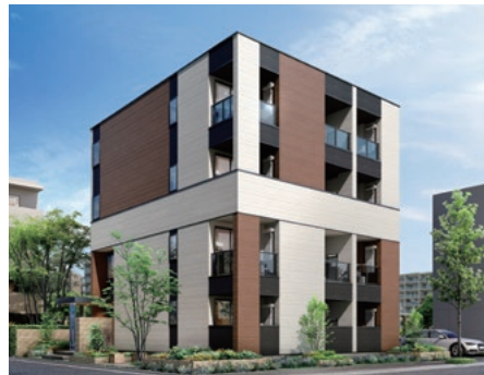
Exterior of Forterb
