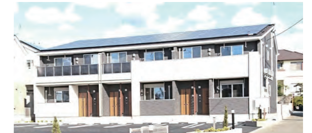
(Izu, Shizuoka Prefecture) Japan's first multifamily rental housing to meet the ZEH standards for detached housing
