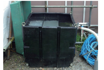
Settling tank installed at a construction site
