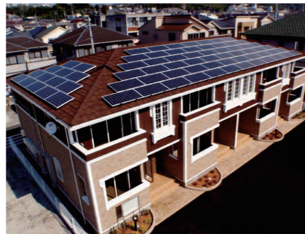
Solar panels generating power on a building managed by the Daito Group
