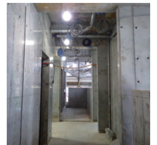
LED lighting at one of our construction sites
