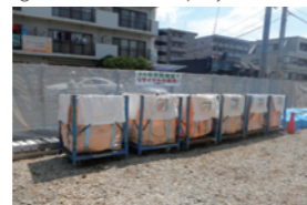
There are 8 sorting categories: waste plastic, waste drywall board, waste wood, other rubble, concrete rubble, waste metal, paper waste, and glass/concrete/ceramics waste
