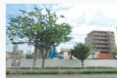
Planned construction site before completion of building
