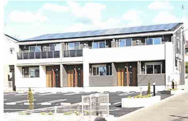
Japan's first multi-unit rental housing project that meets ZEH criteria for detached houses (located in Izu City, Shizuoka Prefecture)
