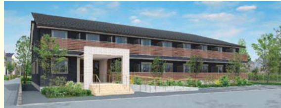
●wooden 2×4 method / all dwelling unit type two-storied (exterior)
