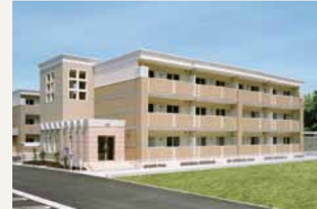
Landule Reinforced concrete
