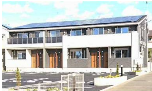
The Daito Group's first ZEH multi-unit housing November 2017, Numazu, Shizuoka
