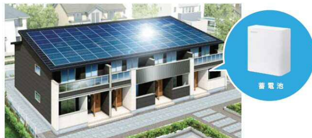
Battery attached, disaster-resilient ZEH rental multi-unit housing On market after June 2021
