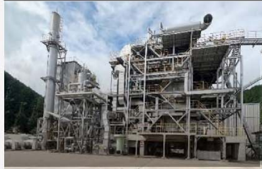
Biomass power generation
